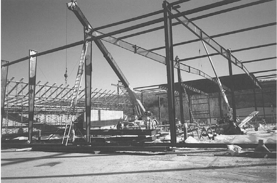
FIGURE 16.1 Assembly of multiple-span rigid frames. The columns at left are stabilized by diagonal bracing and wall girts. (Photo: Maguire Group Inc.)
